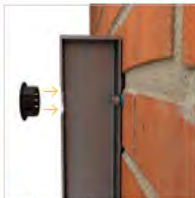
3 Once post is fixed to wall with appropriate fixing method, insert post plug to cover the post hole.
