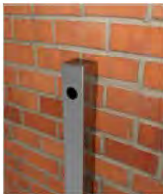
1 Drill a 25mm diameter hole through front wall of post
